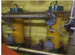
Gambar 3.6: Oil Cooler ( Heat Exchanger ), ( Manual book PT PLN PERSESRO , 2005)
