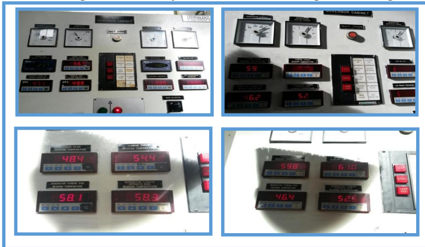
Gambar 4.10 Temperature Turbine Guide Bearing Unit 3 – Unit 6 Normal
